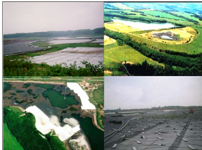
Interim covering on IAA Trünzig B
